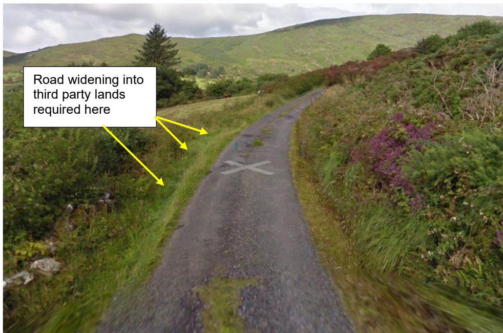
Node 37: Road widening required into third party lands.
