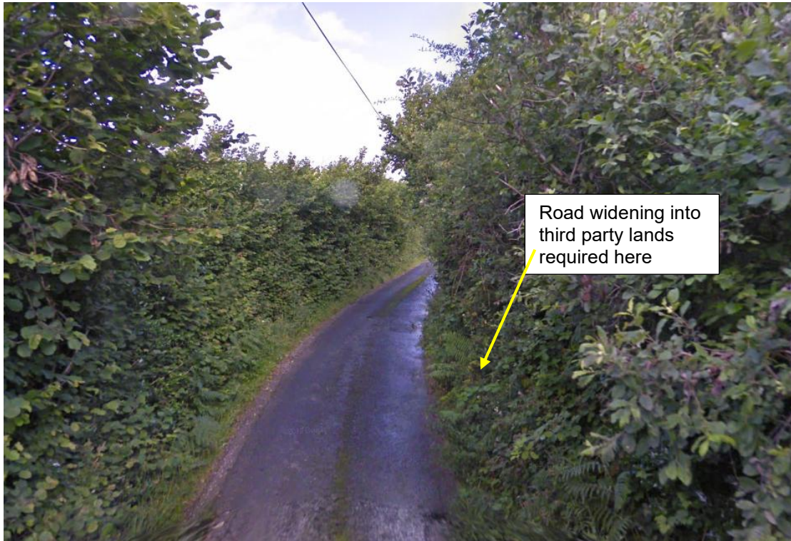
Node 33: Road widening required into third party lands
