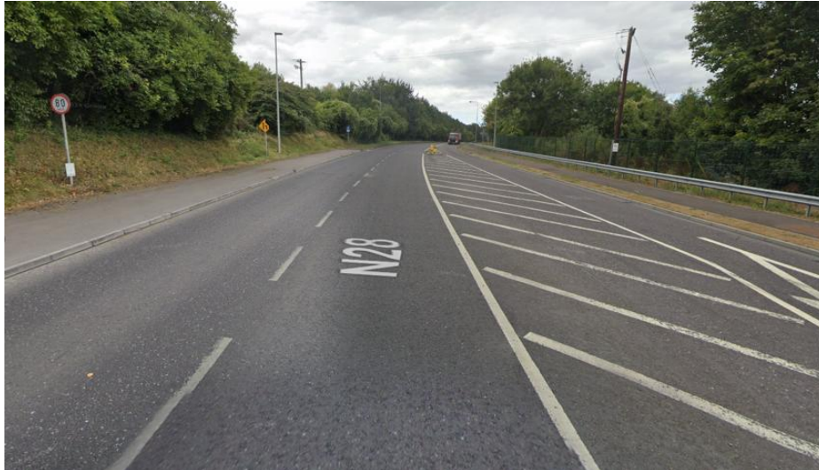
Node 2: N28 westwards from R613 junction.
