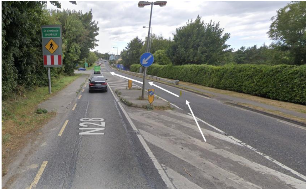
Node 4: Contraflow manoeuvre required around traffic islands.
