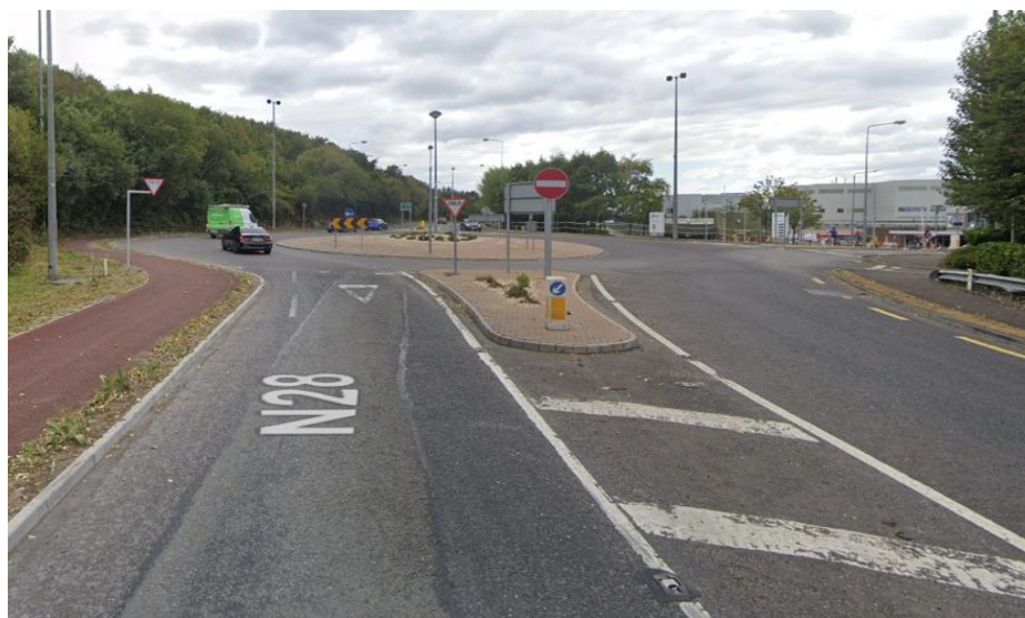
Node 3: Roundabout at Pfizer Factory.
