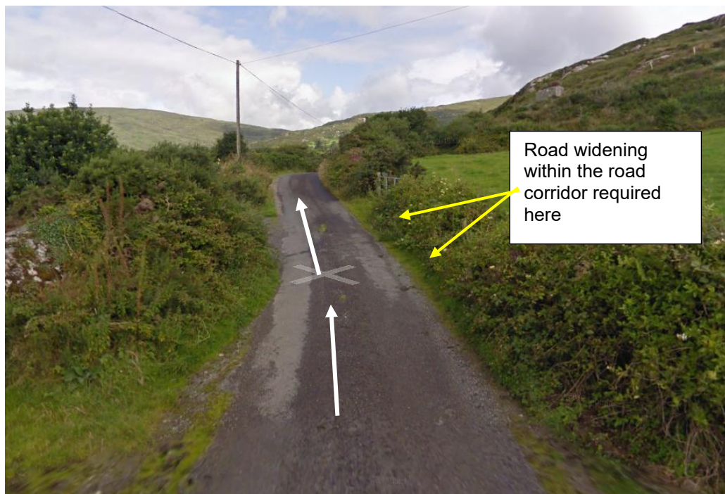
Node 30: Road widening required to the east
