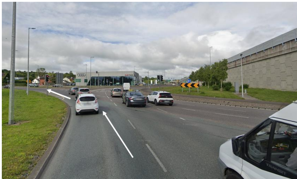
Node 7: Bandon Road Roundabout.
